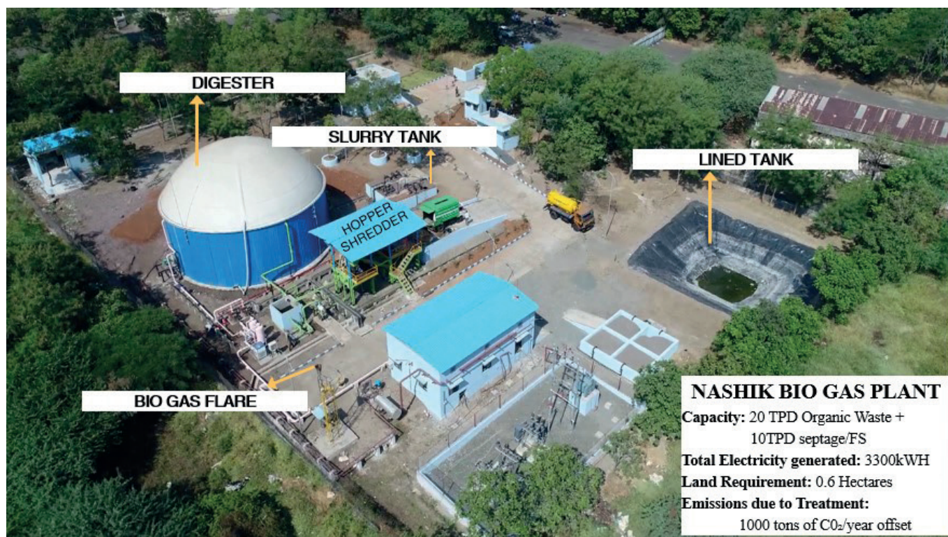
Figure 7: Biogas plant designed by Ecoparadigm in Nashik.
