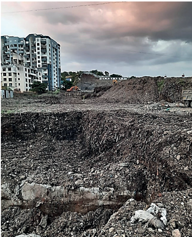
Figure 1: View of the Consolidated Waste
