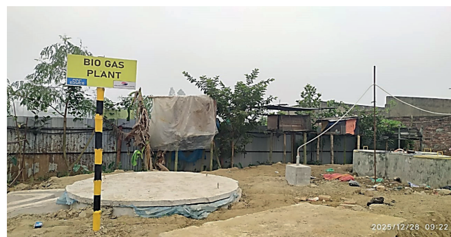
Figure 3: Biogas Plant of DS-08
