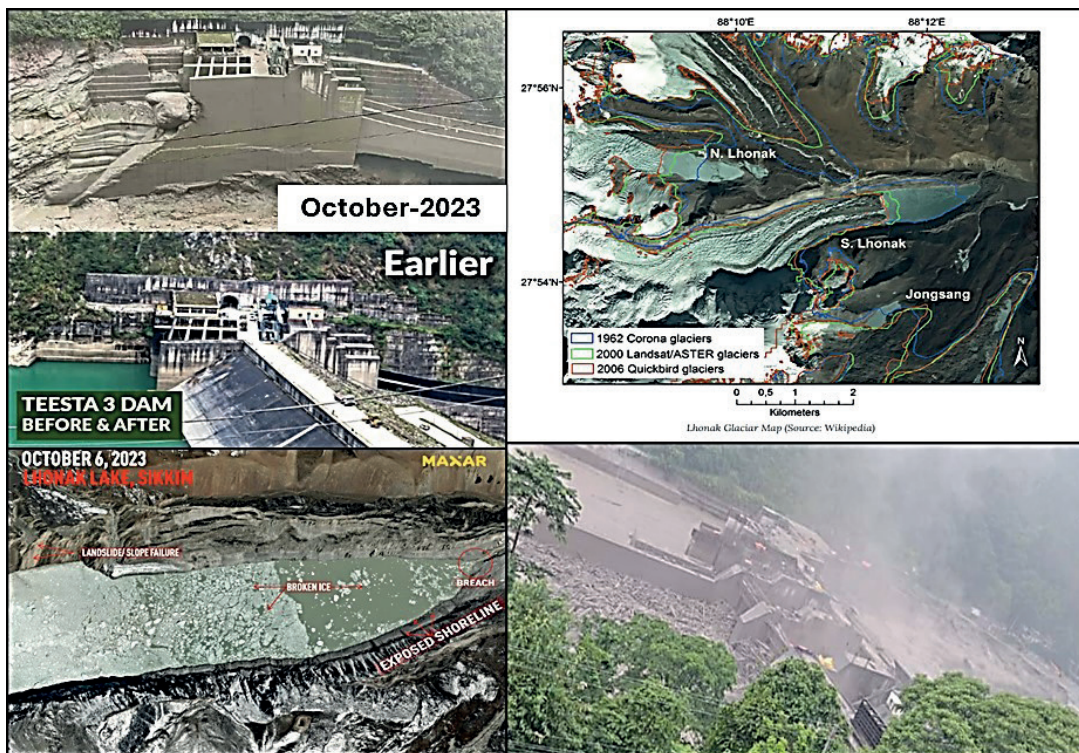
Figure 4: Glacial Lake Flood destroys Teesta-III Dam in Sikkim, brings wide-spread destruction. (Source: SANDRP)
