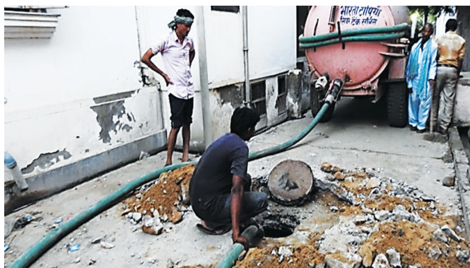
Photographs 1&2: Existing Sludge Collection, Disposal and Treatment in the Pilot Towns
