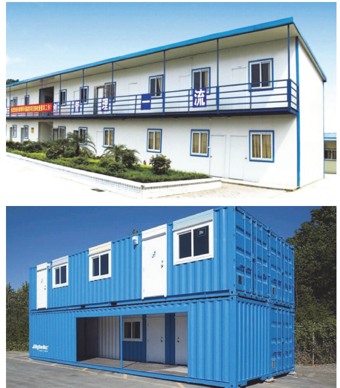
Figure 4: Temporary prefabricated units for construction worker accommodation
