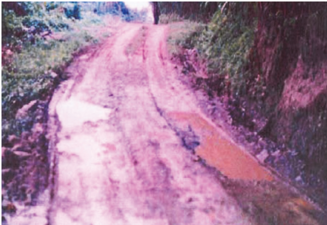
Photograph-3: Washing out of Pavement in a Hilly Road in Mizoram due to Improper Drainage
