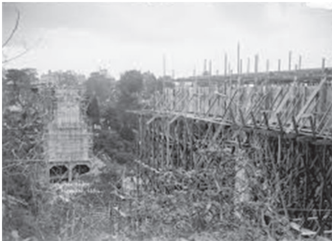
Under construction Grafton Gully, Auckland, New Zealand
