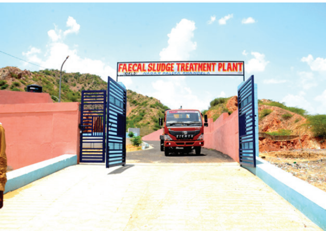
Photographs 4, 5 & 6: Constructed and Operational FSTP in Rajasthan
