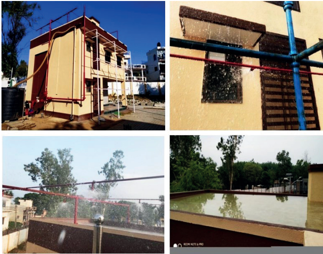
Figure- 5: Full-Scale Test for Water Tightness on RC Precast Component Building
