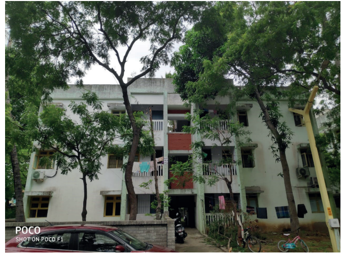
Figure-3: G+2 Floor Apartment
