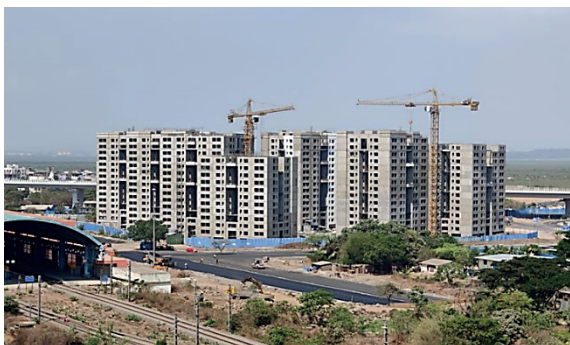
CIDCO Kharkopar site deploys Pre-Cast construction technology
