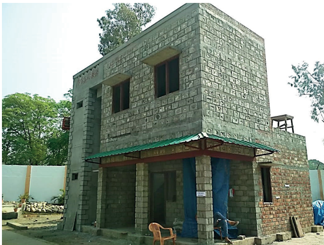
Figure-4: Round Boulder Units Confined Masonry Building
