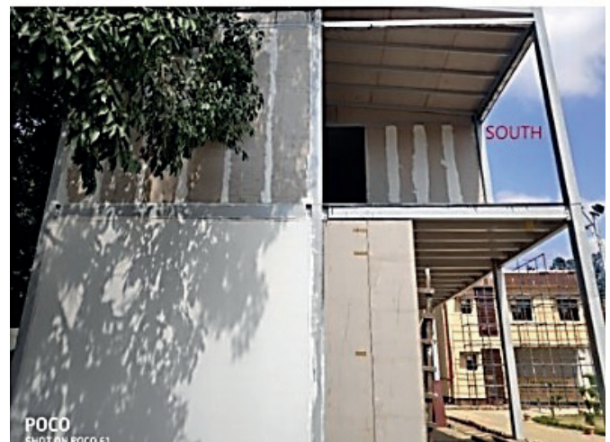
Figure- 2: Steel building with light-weight infill panels
