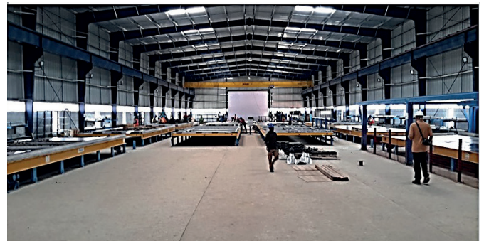
Carousel Plant at New Haven, Peenya, Bangaluru, Tata Housing
