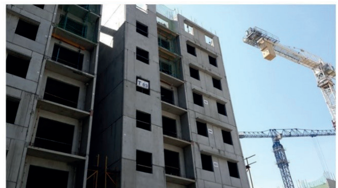
Precast construction - under erection at Peenya, Bangaluru – Tata Housing
