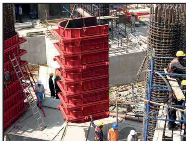
Pre-engineered formwork
