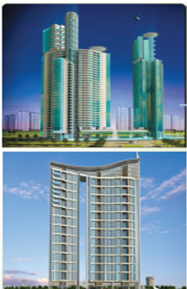
Figure-3. Some Typical Tall Building Images of Unconventional Geometry
