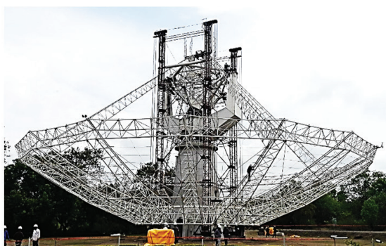
Antenna Dish lowered to the Ground Position on 17 th June 2022
