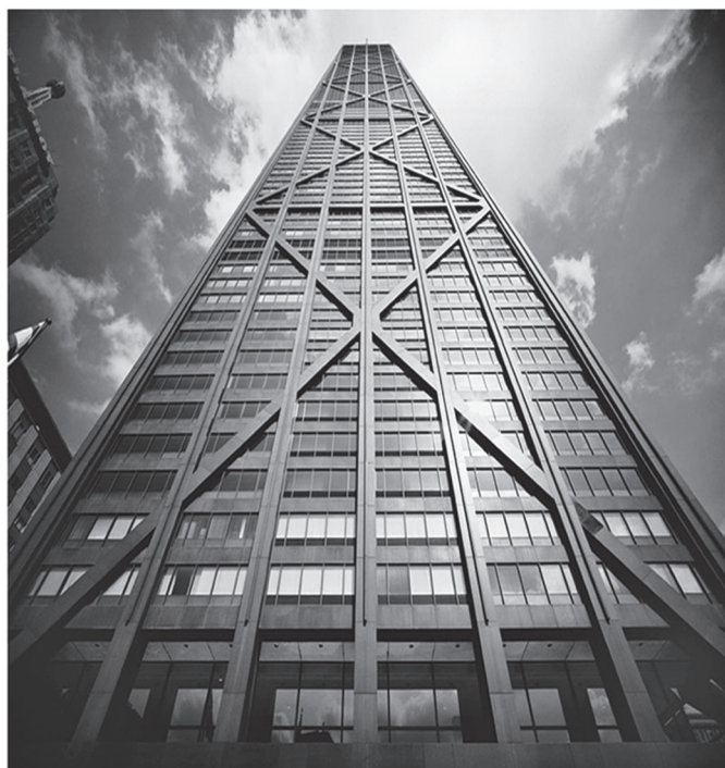
Figure-10: Bracings at Peripheral Facade
