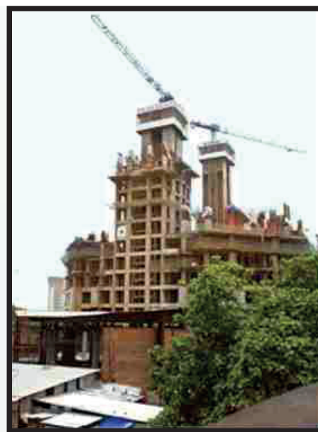
Automatic climbing formwork for cores
