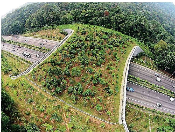
Typical view of Eco-duct / Animal Overpass
