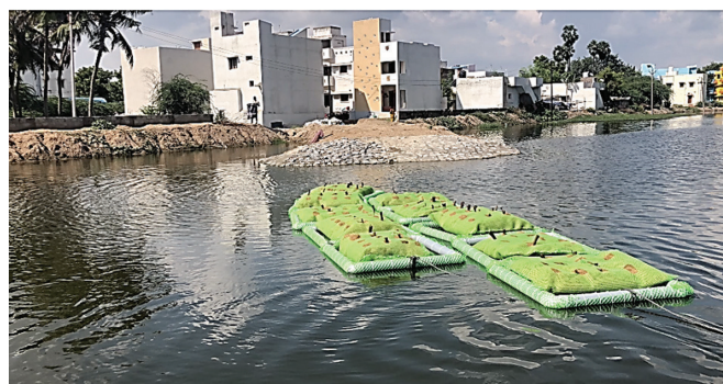
Floating wetlands absorb the nutrients in the wastewater
