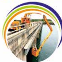
Bridges, Flyovers, Interchanges and Other Structures
