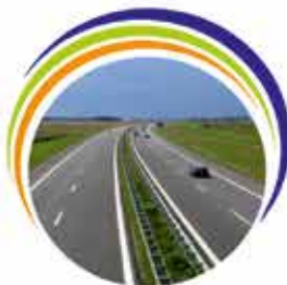
Expressways, Highways and Roads
