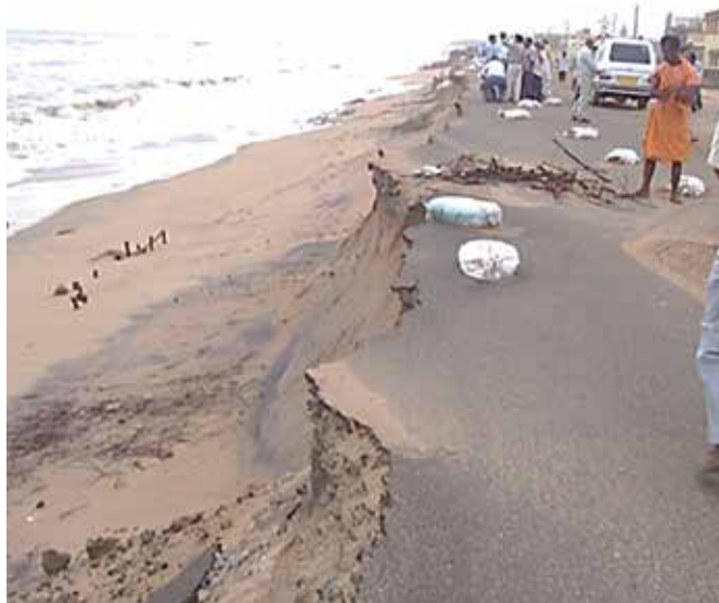
Photo-1: Erosion at Puri in between Lighthouse and Sterling Hotel beaches
